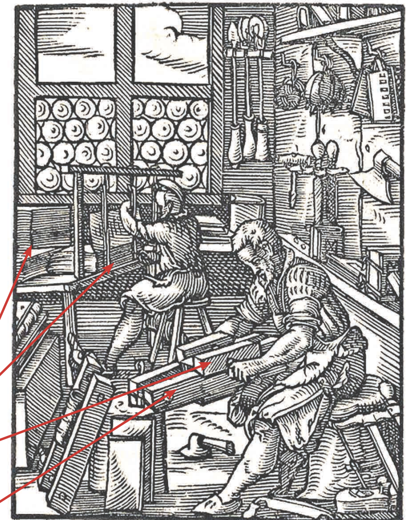
Figure 4. Jost Amman's 1568 woodcut from the Book of Trades graphically demonstrates the use of the plow, trimming the edge of sewn signatures held firmly in a heavy wooden clamp. Like the deckle, the back mark of many quarto and octavo folded books may have been trimmed or partially trimmed off in this step.
